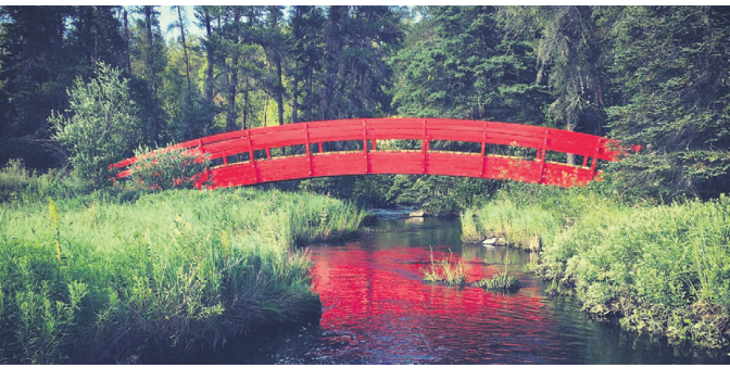
Refurbished bridge relocated from King's Park in Winnipeg allows Trail users to cross Hanson's Creek in Whiteshell Provincial Park in Manitoba. TIM COFFIN
