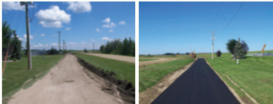
The Lacombe County Trail, before and after paving.
