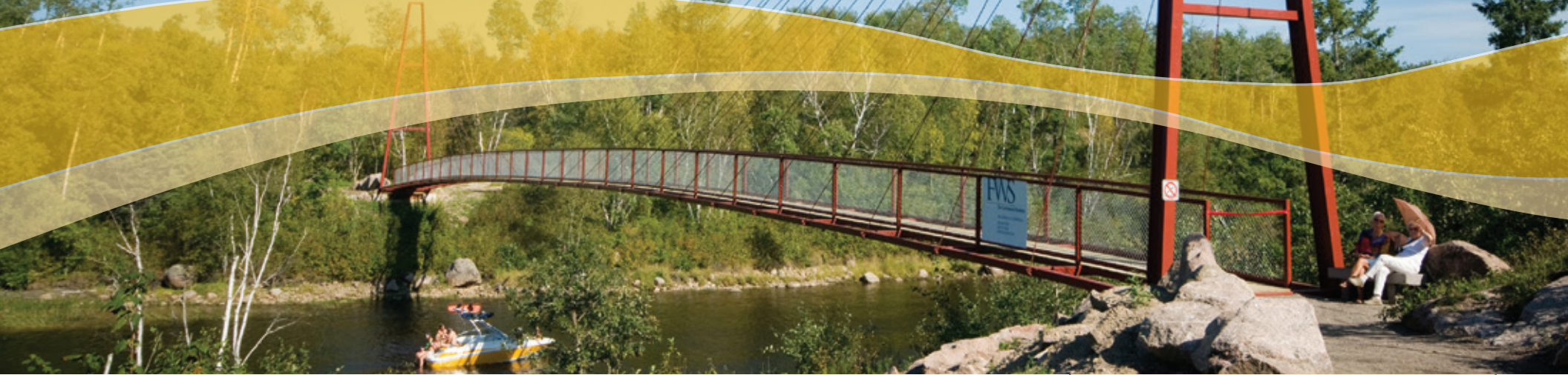
Whiteshell River Bridge on the Border to Beaches Trail in Manitoba. Photo: D. Lipnowski, Trails Manitoba.
