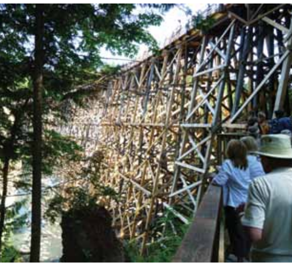
Kinsol Trestle Grand Re-opening, July 28 2011 (photo: Ingrid Vermegen)
